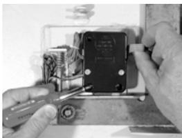
3. Using two of the 1/4-20 (or M6) screws in the kit, loosely attach the lock body to the safe's mounting plate. This is just to hold it in place during cable attachments to the keypad and keypad extension. Be very careful to avoid crushing or crimping the cables. Note the black/red/green wire bundle. This is for the *bolt position*
